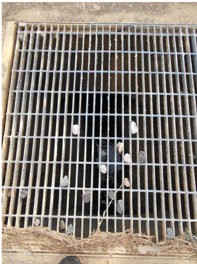
Plate 7.2 Drain set into base of the drainage channel, with water visible in the base of the drain.
